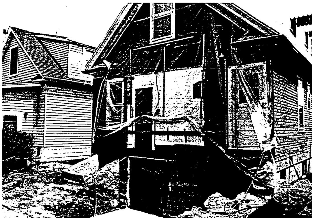
Fig. 4. View of back of house at 90 Avenue C where kitchen and steps to basement have been removed.
