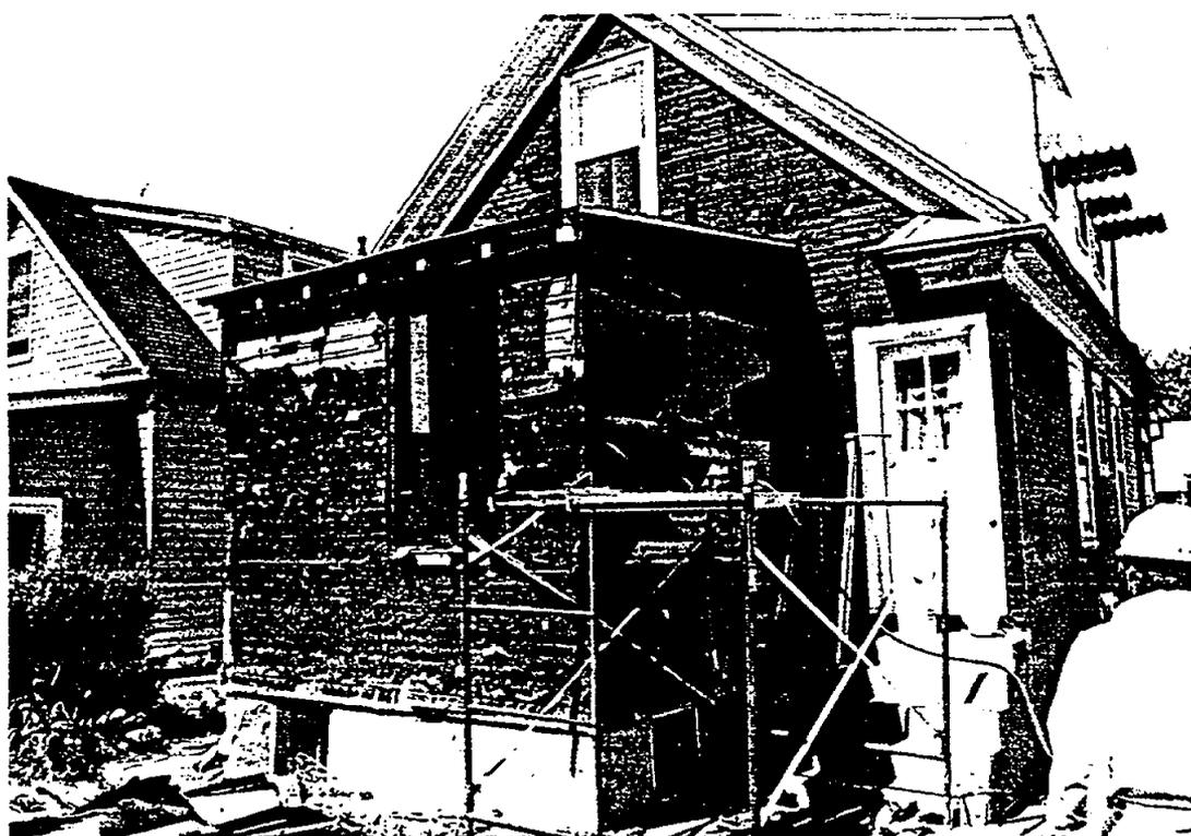
Fig. 3. View of the back of the house at 90 Avenue C, Lodi, New Jersey, being remediated. Kitchen and steps to the basement and are being removed.
